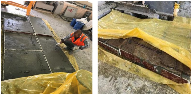
Fig. 3 Concreting and curing the slabs.
